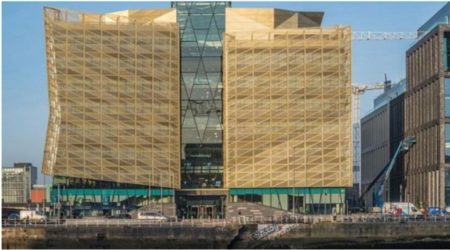
The Central Bank on North Wall Quay in Dublin has won national and international awards for its accessibility.
